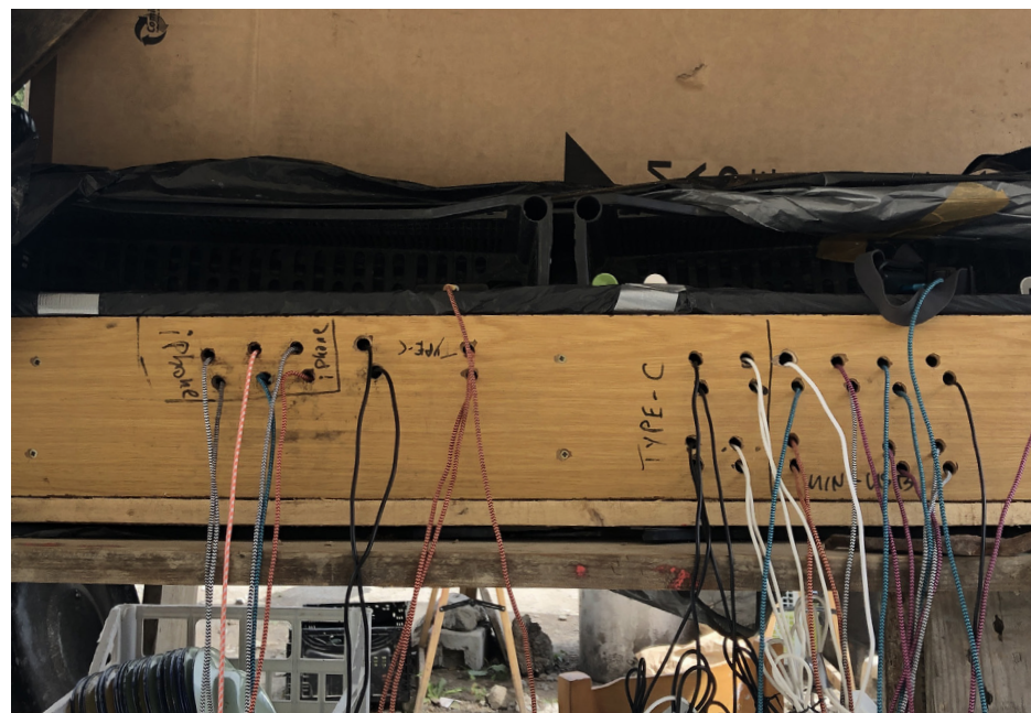
charging station operated by the solar system
